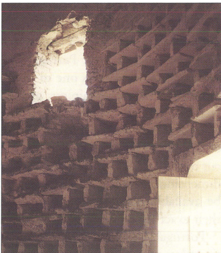
FIG. 8 The interior view of the large window and of the narrow door, showing another set of nesting-niches. The total number of nests is 872.
