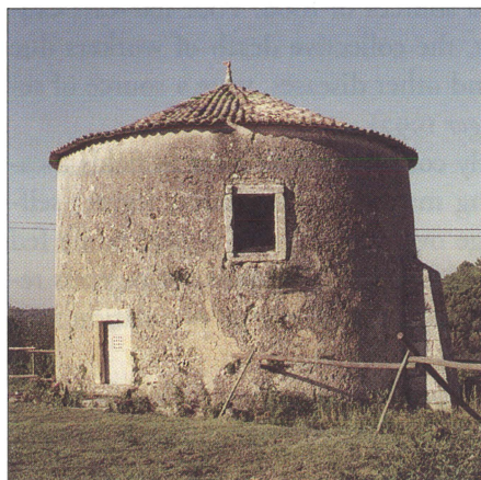
FIG. 3 The dovecot from the XVI century is an independent circular building built about 70 meters from the cloister. The door faces south west and the large window faces south. The height of the dovecot is 7.70 meters and its external diameter 7.76 meters.
