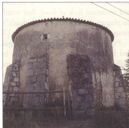
FIG. 4 The dovecot photographed from the opposite side showing the four ramparts built to preserve its structure. The small window facing east is seen at the top.
