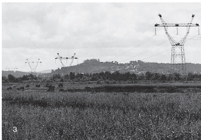
Figure 3. General view of four high-tension poles, all having white stork nests.
