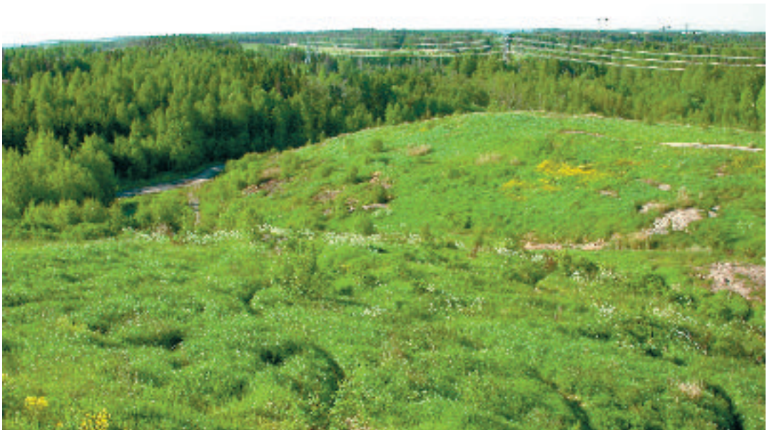
Figure 1. Different parts of the Vuosaari landfill. Upper left: The northern part of the heaping mound in the early stage of landscaping on 24 April 2004. Upper right: The eastern side of the landscaped heaping mound from the north southwards to the Vuosaari harbor on 9 June 2005. Lower left: A northeast view to the heaping mound over the bushy habitat of, among others, the Whinchat Saxicola rubetra and Common Grasshopper Warbler Locustella naevia in the middle part of the old landfill on 26 May 2004. Lower right: A southwest view of the bushy grassland of the southern part of the old landfill on 9 June 2005. All photos © Tapio Solonen.
