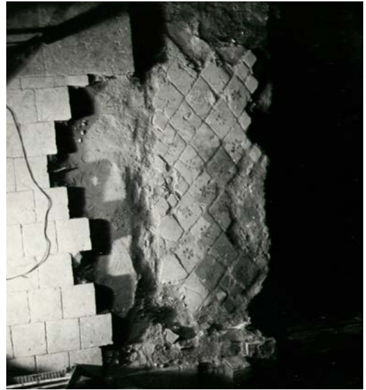
Fig. 4. A small part of the oldest floor of glazed tiles from the abbey Church of Sorø, found in situ in front of the steps into the main chancel. The tiles show traces of fire from burning roof beams which had fallen from the roof. Photo: H. Stiesdal 1970, the National Museum.
