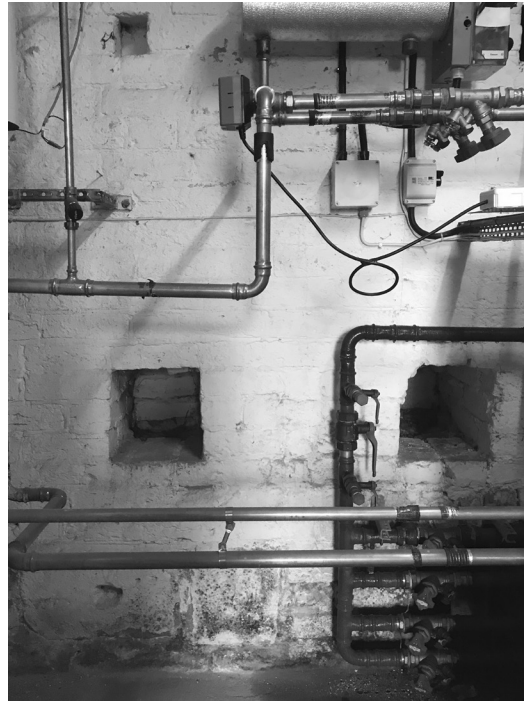
Fig. 4. The holes in the cellar wall indicate a demolished wooden floor. The cellar was once much deeper before it was drowned when the mill was moved downstream and the water level in the river was raised (photo by Anders Ödman).
