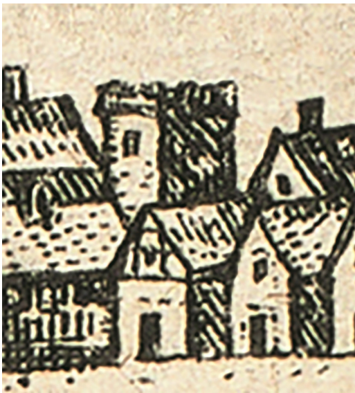
Fig. 13. Tower house in Lund, maybe the main building of the Bille Manor. Source/photo by Lund University Library, Alvin item no. 76516.
