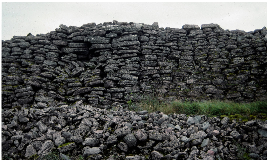
Fig. 9. Gråborg: Part of the secondary inner wall. Note the vertical joints, the building technique and the part of the wall where stones are disturbed (or have fallen down?). Photo by G.Malm 1997-2002.
