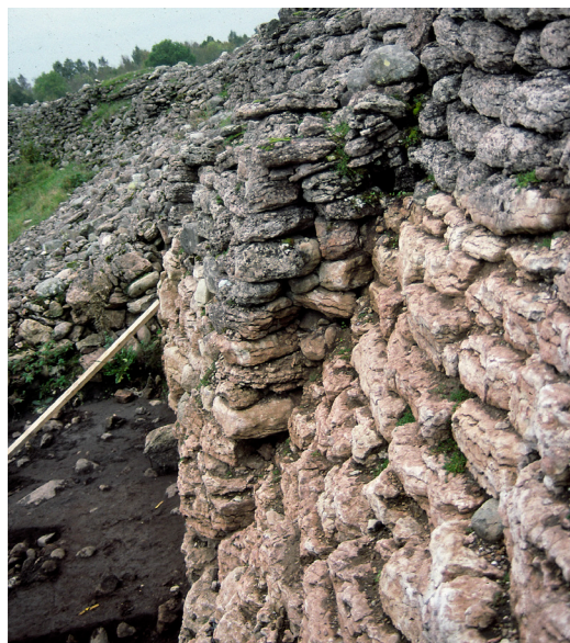
Fig. 7. Gråborg . The secondary inner wall leaning against the stepped inner side of the high wall. Beyond you see the heap or row of stones against the inside of the wall. Photo by G. Malm 1997-2002.
