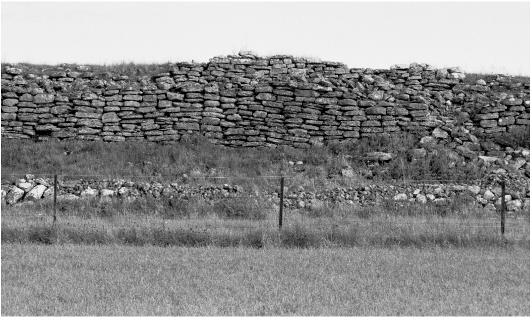
Fig. 10. Part of the secondary outer wall. Compare the building technique and the vertical joints with the secondary inner wall, figure 9. Photo by G. Malm 1997-2002.
