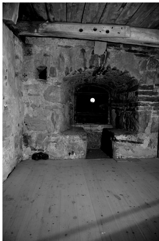
Fig. 13. One of the windows in the west gable of Room 2 (401), with the local limestone in the embrasure, photographed from the east. Photo by T. Westergren 2011.
