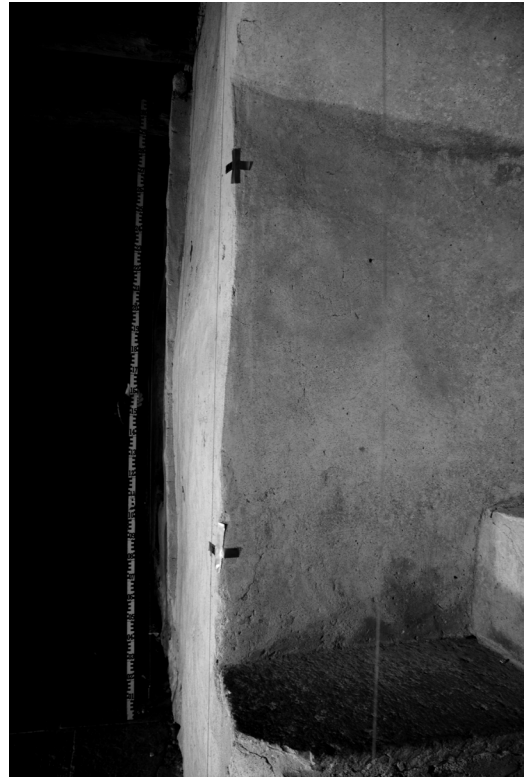
Fig. 7. The easternmost of the vertical courses on the north wall of Room 1 (301) photographed from the east. Photo by T. Westergren 2011.
