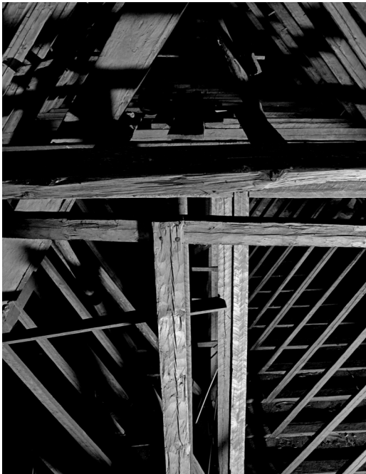
Fig. 6. The roof trusses above the nave in Bredestad. Notice the sprättäljning on the suspended beams, apparent in the oblique lightning. Photo by R. Gullbrandsson.
