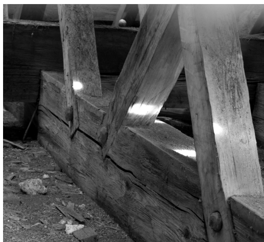
Fig. 4. Detail of tie beams above the chancel in Norra Solberga with wooden pegs shaped like nails. Photo by R. Gullbrandsson.
