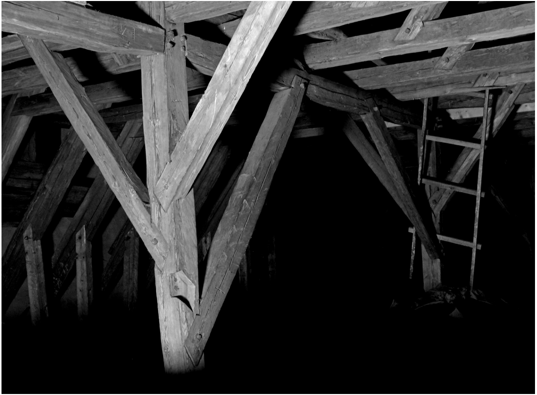
Fig. 14. Detail of the roofing in Askeryd with the lower part of two king posts. Photo by R. Gullbrandsson.
