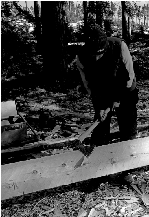
Fig. 11. Carpenter Mattias Hallgren, Traditionsbärarna, cutting boarding for the reconstruction of Södra Råda church, using the technique of sprättäljning . Photo by R. Gullbrandsson.
