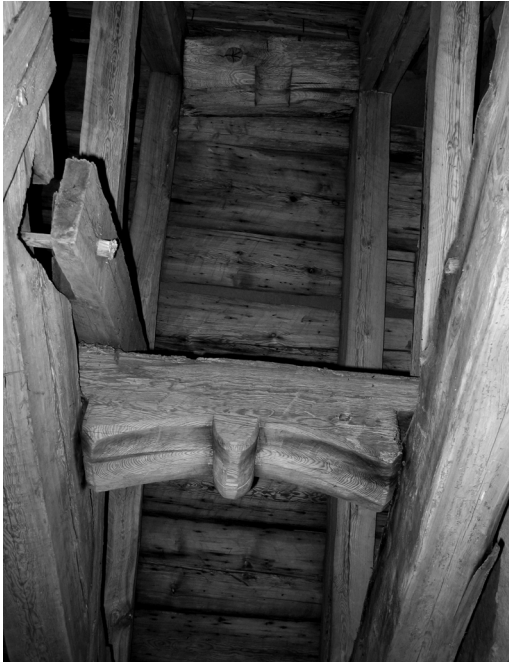
Fig. 8. Decorated steering plate and ridge purlin in Bälaryd. Photo by R. Gullbrandsson.
