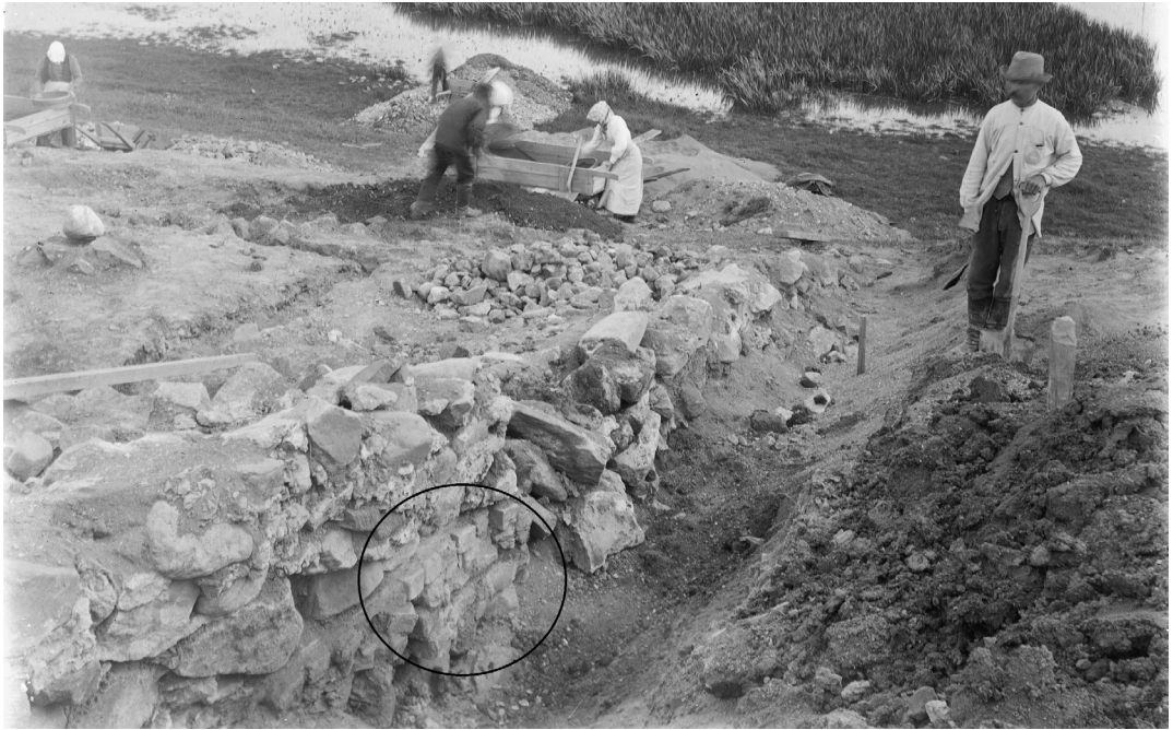
Fig. 8. Foundations of the of the eastern masonry building from the north-west. Note the bricks in the structure. Photo by J. Ailio, Museum Centre of Turku.
