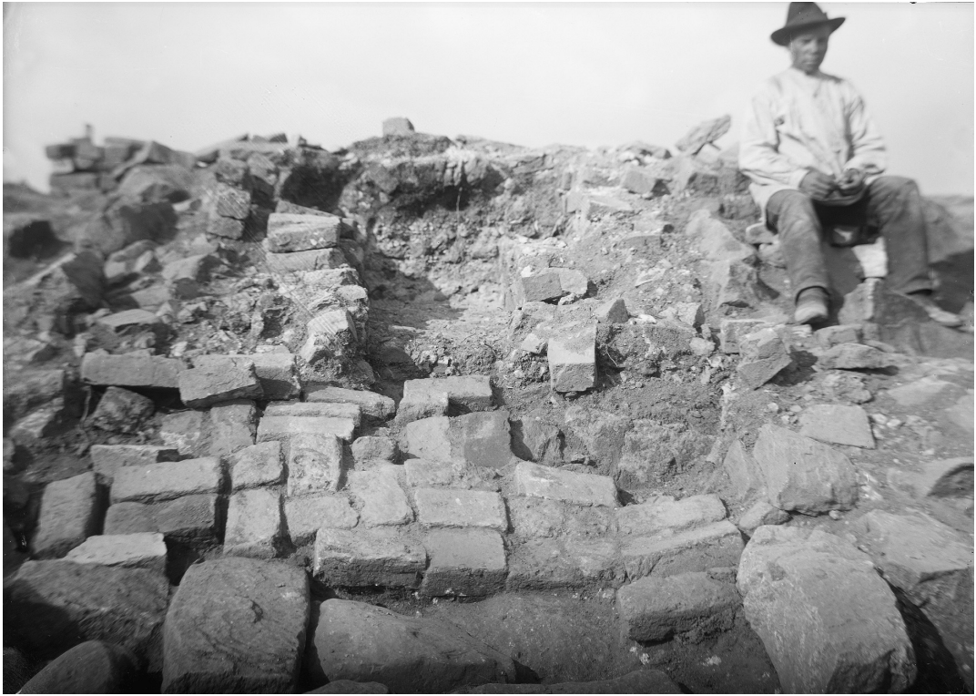
Fig. 11. Heat-storage hypocaust from the south. In front the remains of the brick floor. Photo by J. Ailio, Museum Centre of Turku.
