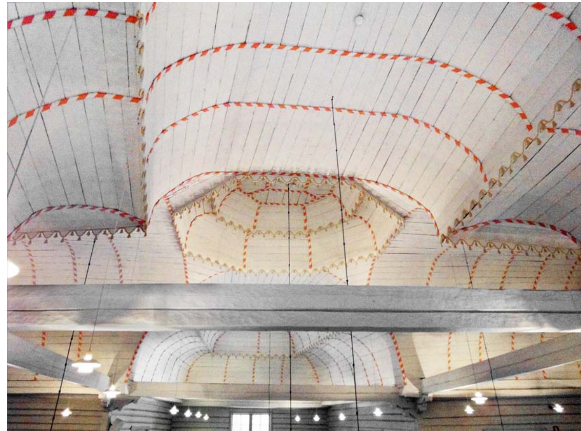
Fig. 27. The ceiling in the church of Lemi. The octagonal recess marks the crossing. The trefoil section of the cross-arm ceilings, which is seen in the background, is a sign of Gothic survival. The lambrequins and the decoration in red are original ornaments, but painting the surfaces of the vaults white may date from 1874 when the entire interior was painted, possibly for the first time. Photo E. M. Viljo 2016.
