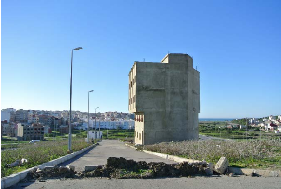
Buildings, Tangier, 2017. Photo: Eugénie Denarnaud.
